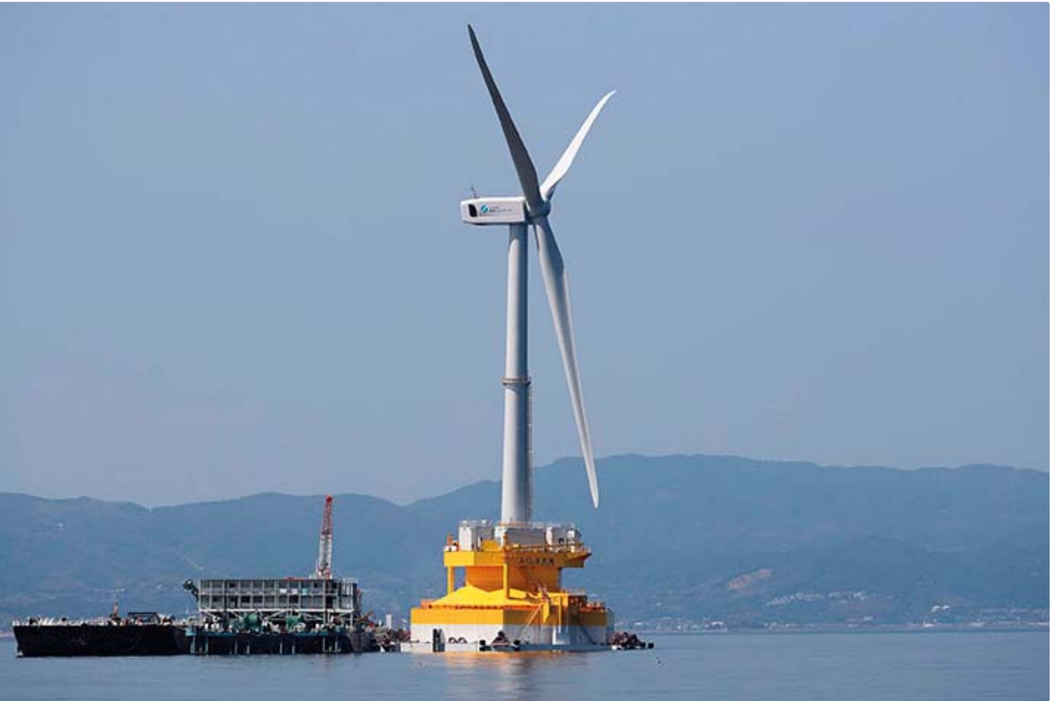
Hitachi 5MW floating offshore wind turbine © FukushimaFORWARD
