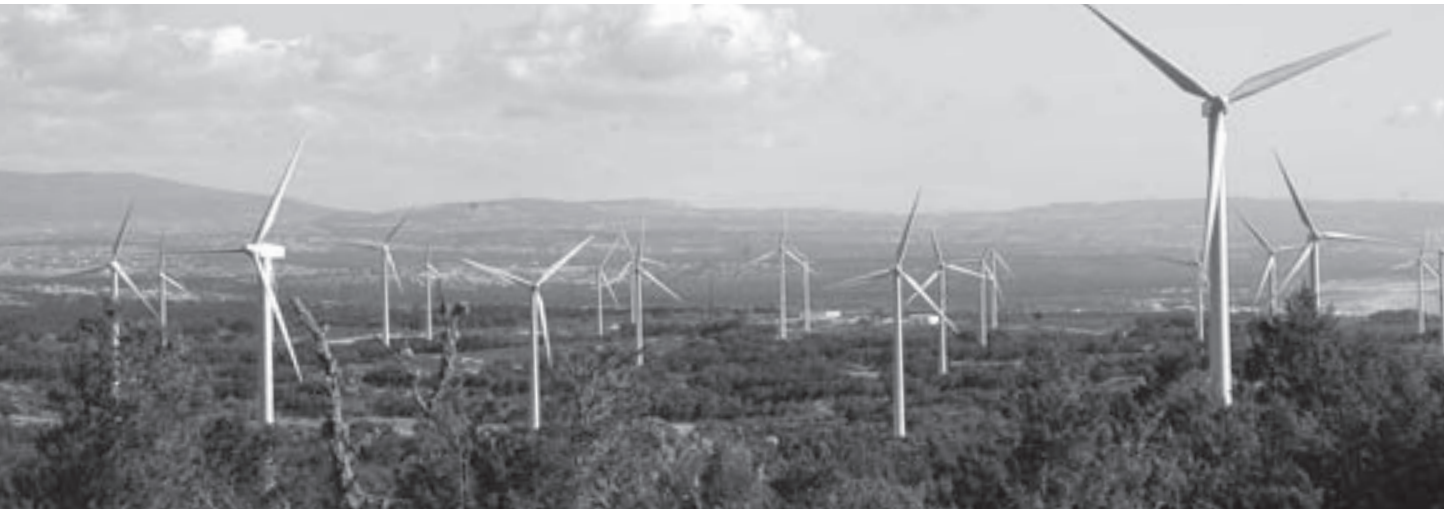
Amogdoul wind farm, Morocco
