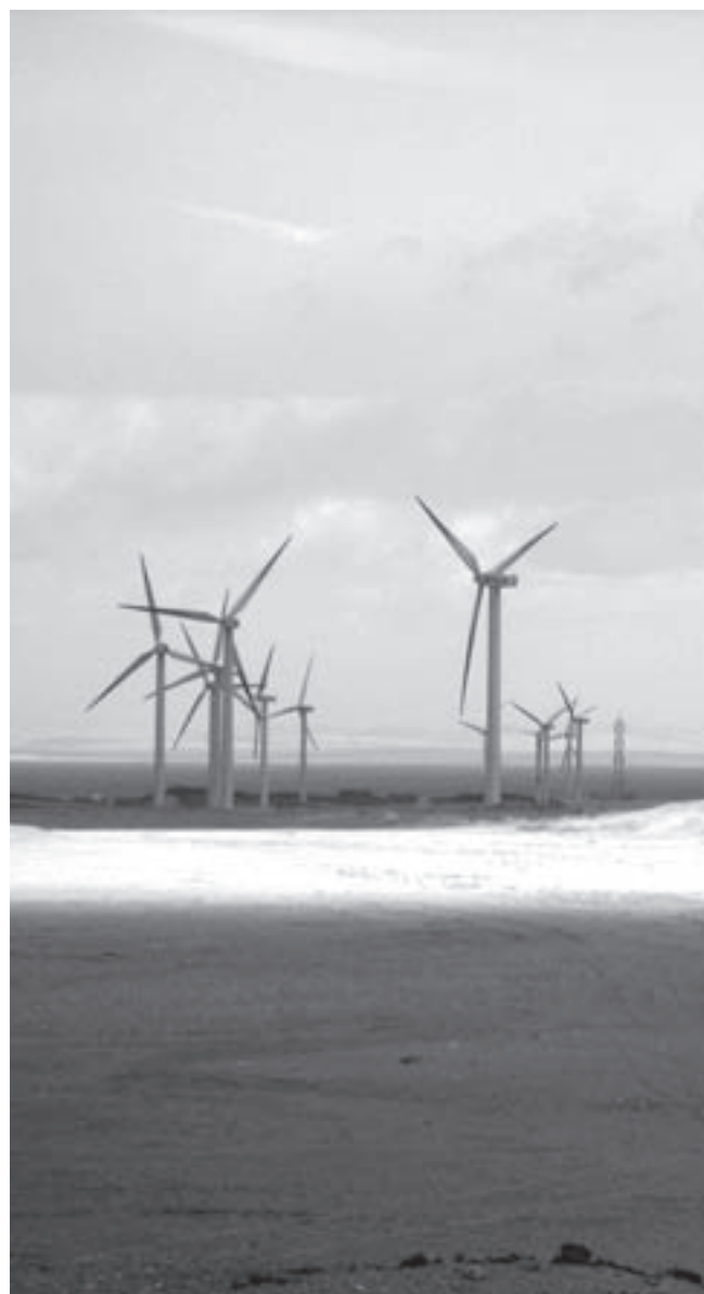
Zafarana wind farm, Egypt
