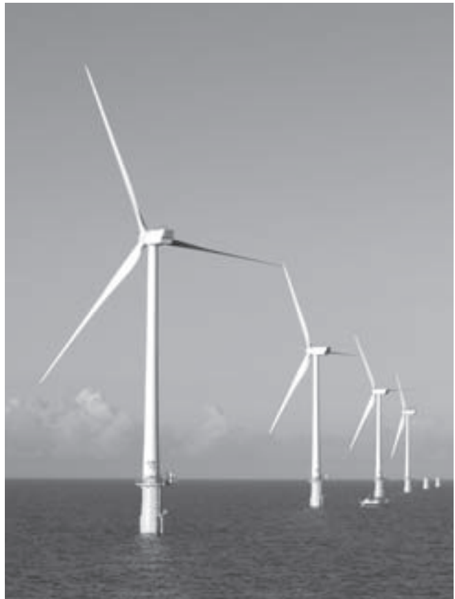
Barrow off-shore wind farm, UK
