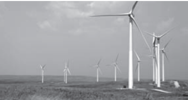
Soderglen wind farm, Southern Alberta, Canada
